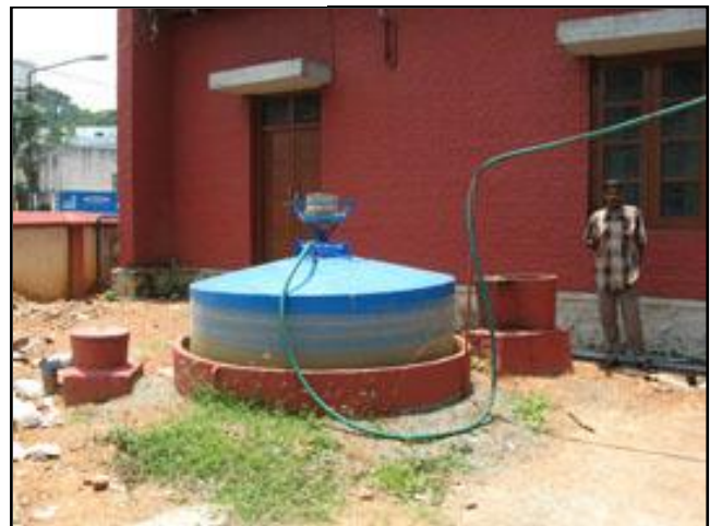
Figure 2. Digester for treatment of feces and kitchen waste in Trivandrum, India. Photo courtesy of Eawag.
